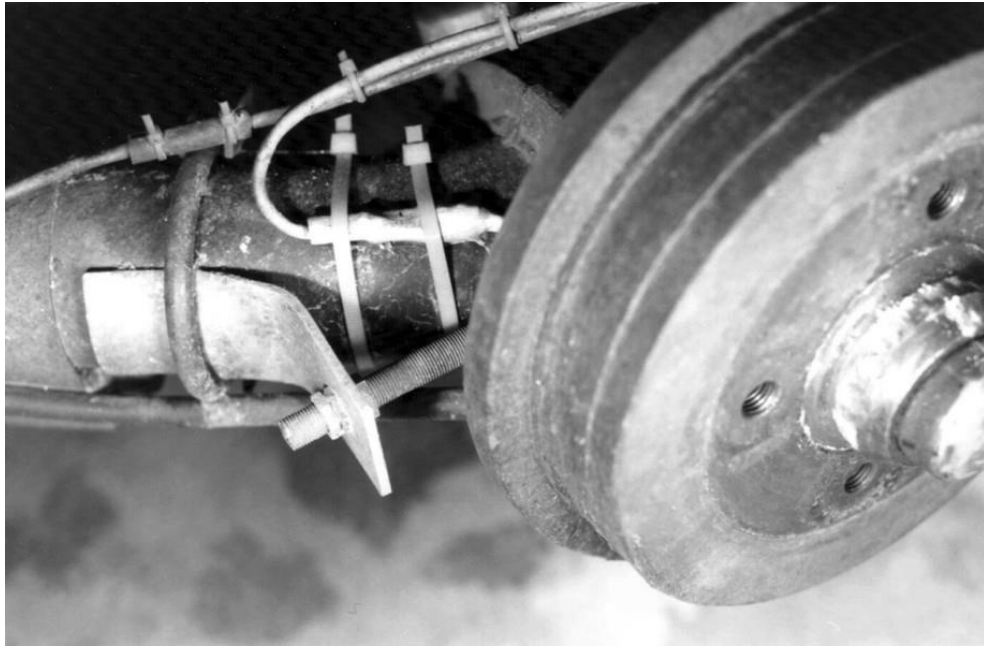
Figure 13-7: A wheel-mounted transducer installation
